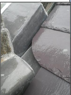
The completed high level roof with its new Welsh slates is impressive.
